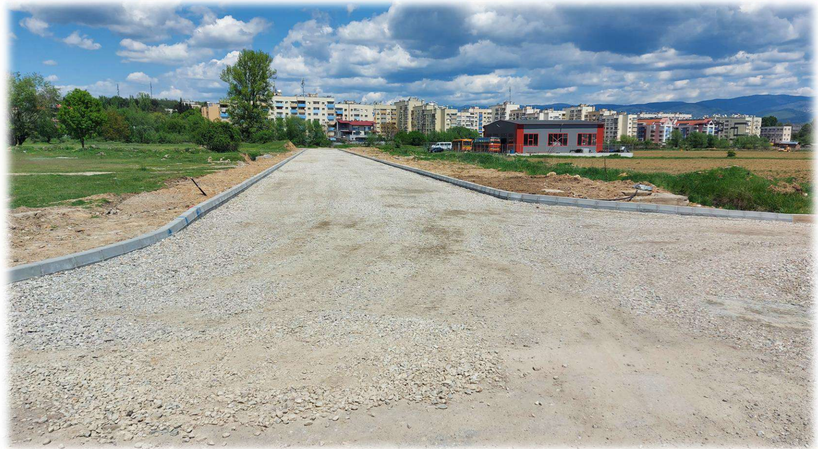
Construction of a ring road to relieve traffic in the center
