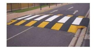
The solution adopted is to create speed moderation works also on these extra-urban roads by introducing raised crossings and luminous signs
